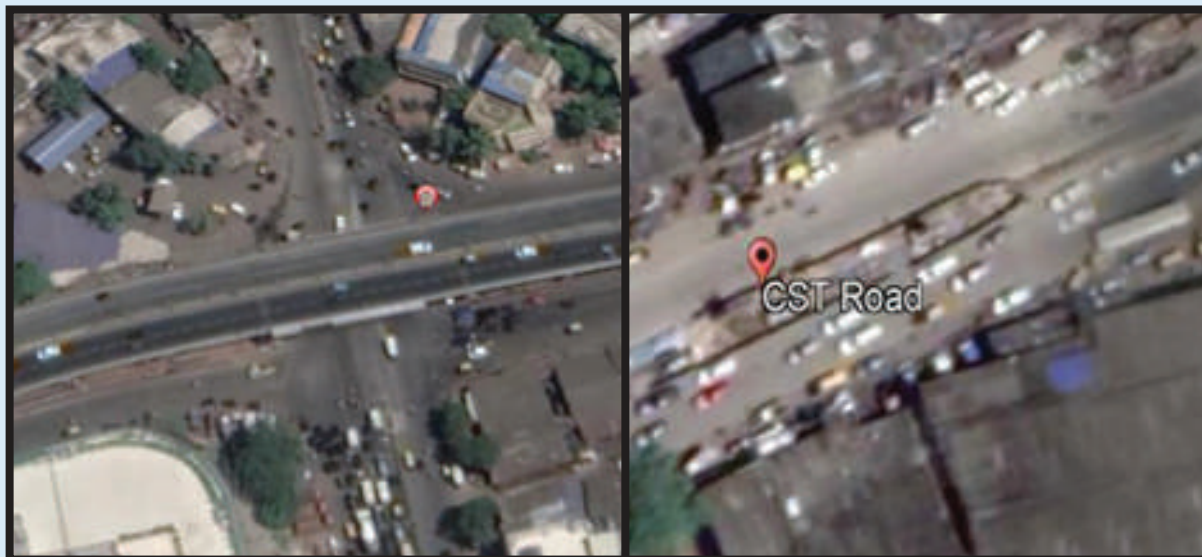
Figure 19: Google earth view of CST Bridge, near Kurla Bus Depot, Kurla West
